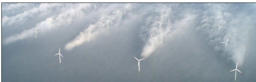
Figure 8.15 The 'wake' effect created by wind as it goes past one generator affects other generators down the line, decreasing the expected power output of the windmill 'farm'.
